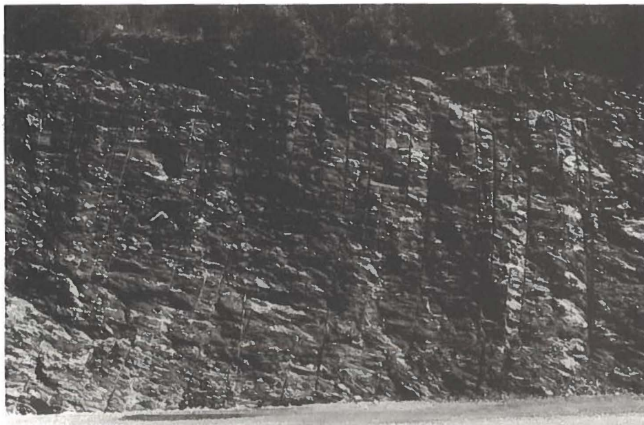
Photo 2. Bulken (Norway). Typical slant layered rock with up-dip unidirectional hole deviations. [Photo Thomson Sinkala]
