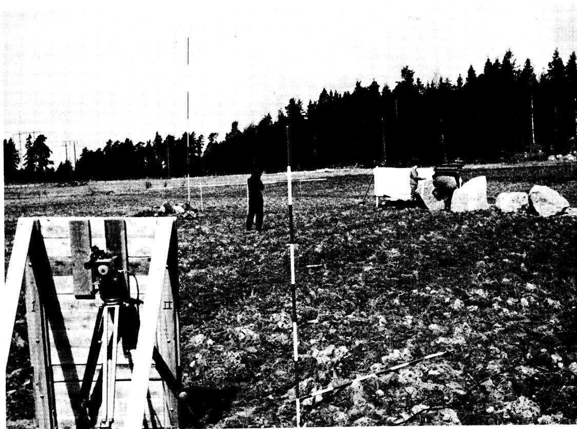
Fig. 4. Arrangement at bench blasting.
