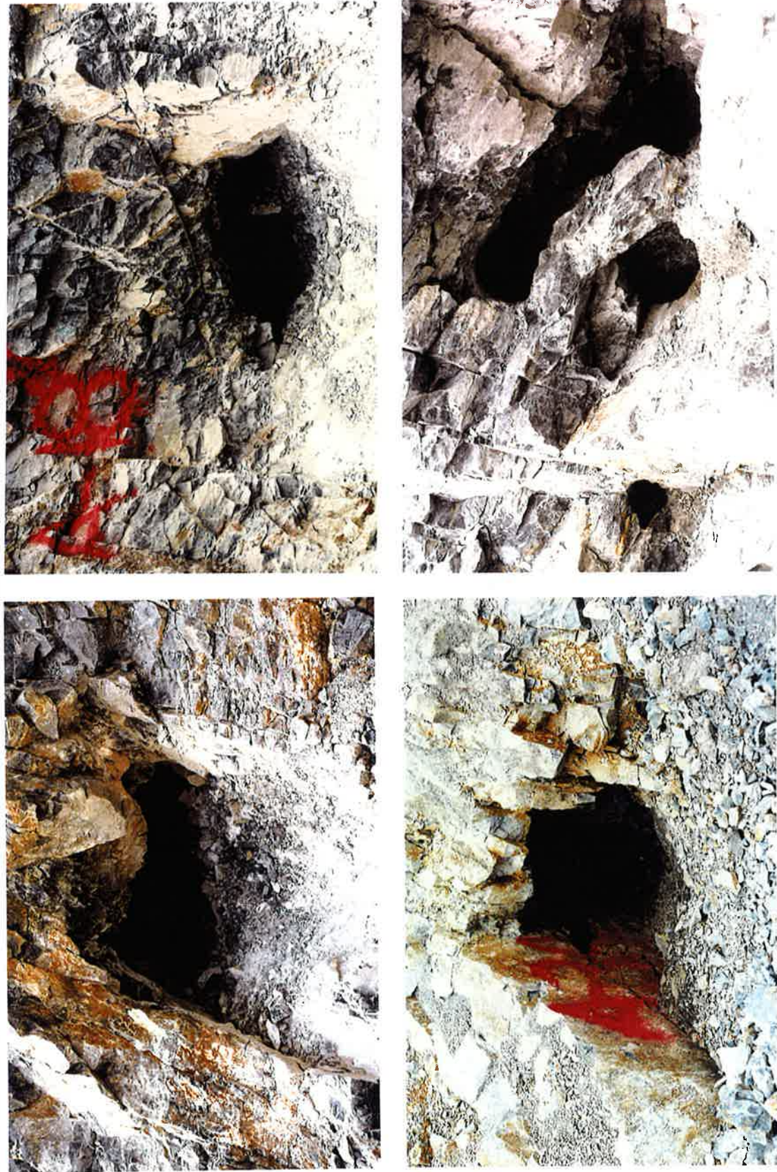
Figure 17: Post-blast photos of cuts; top row A-20 (new A-4) & A-18" (new A-20), bottom row A-34 (new A-1) & A-12 (new E-6).
