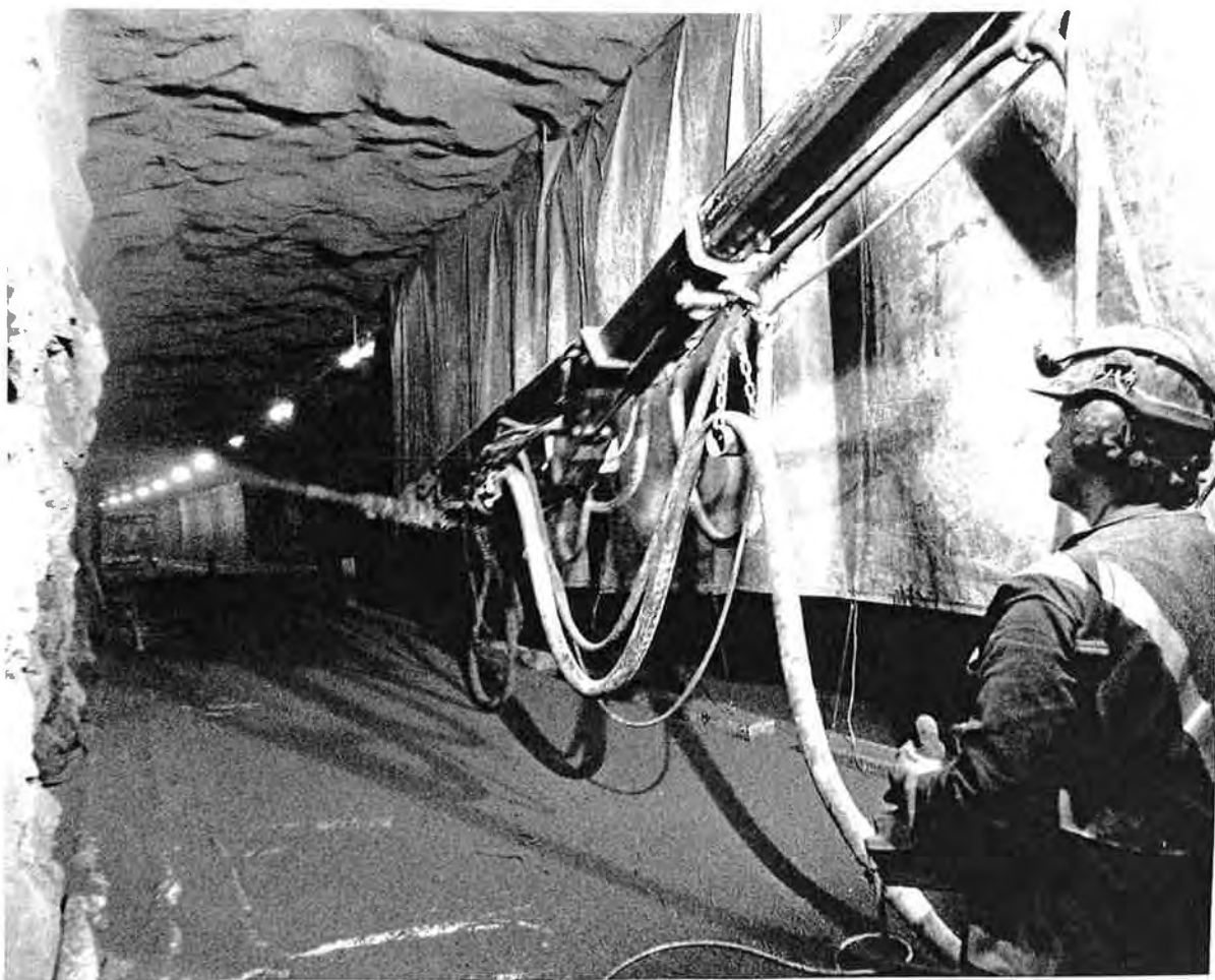
Figur 9 Betongsprutning Shotcreting
