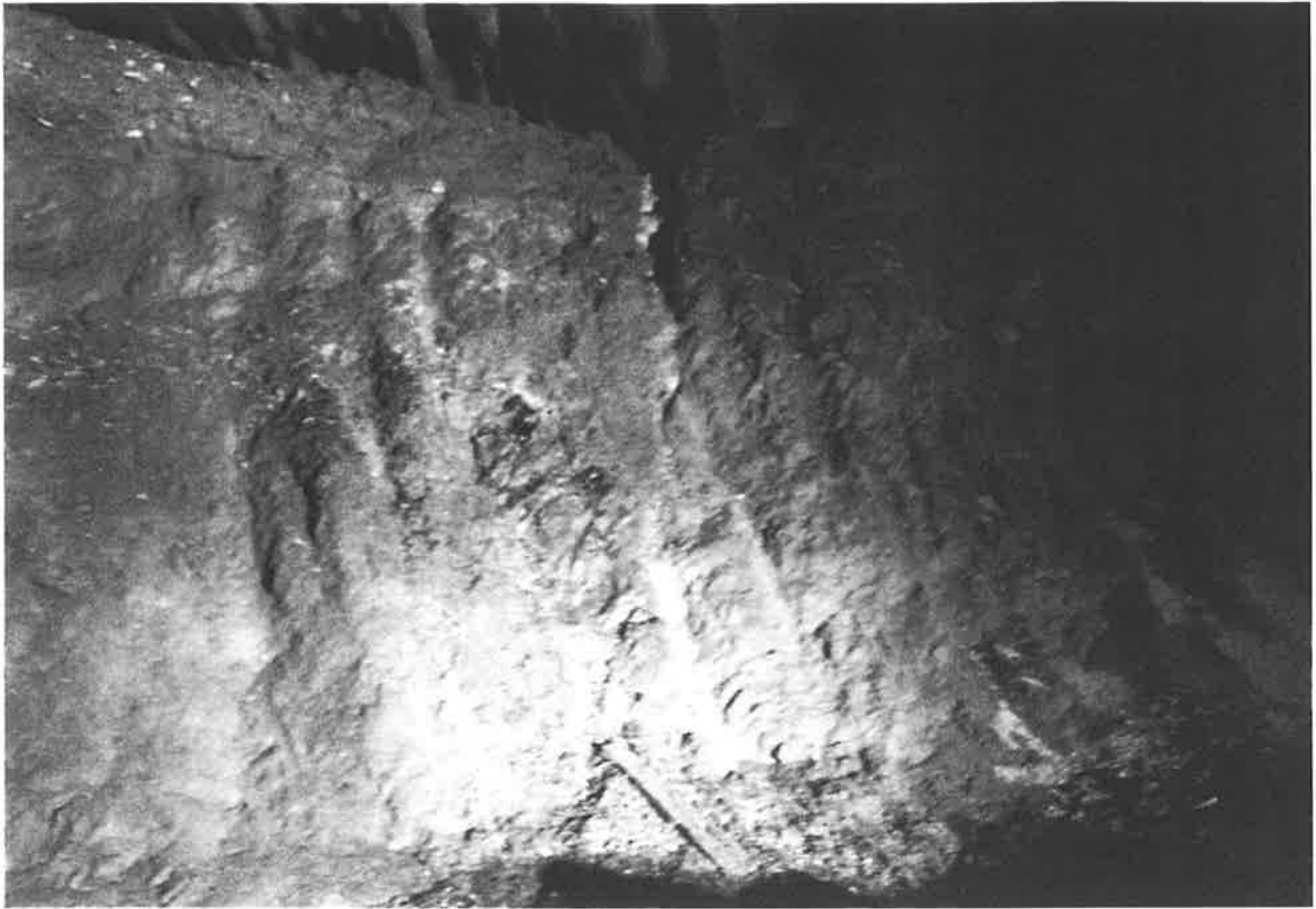
Figure 3.1 The rock was soft enough to be excavated by excavator. View of the bench.
