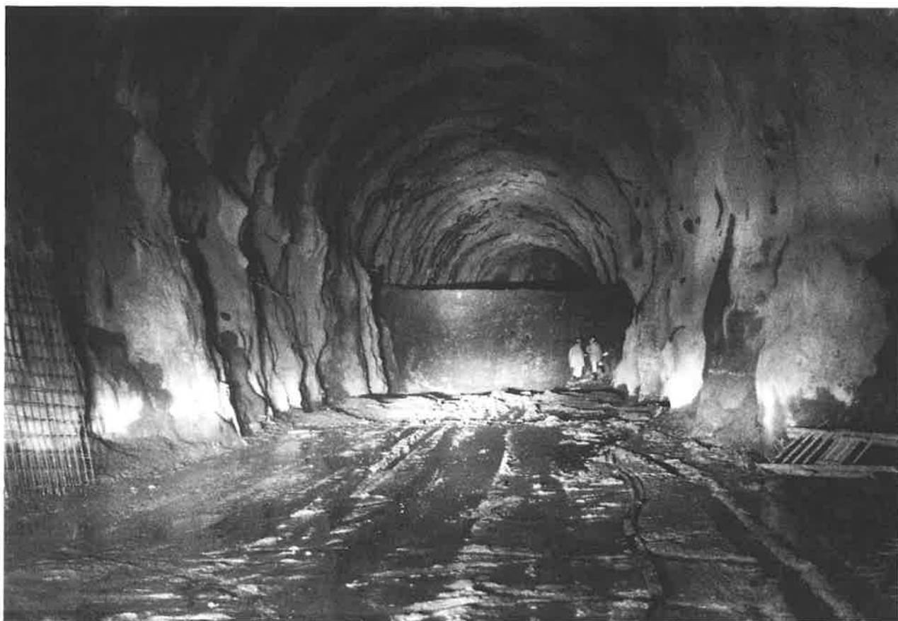
Figure 3.2 The tunnel was excavated by multiple drift. View towards the bench and the divided heading.
