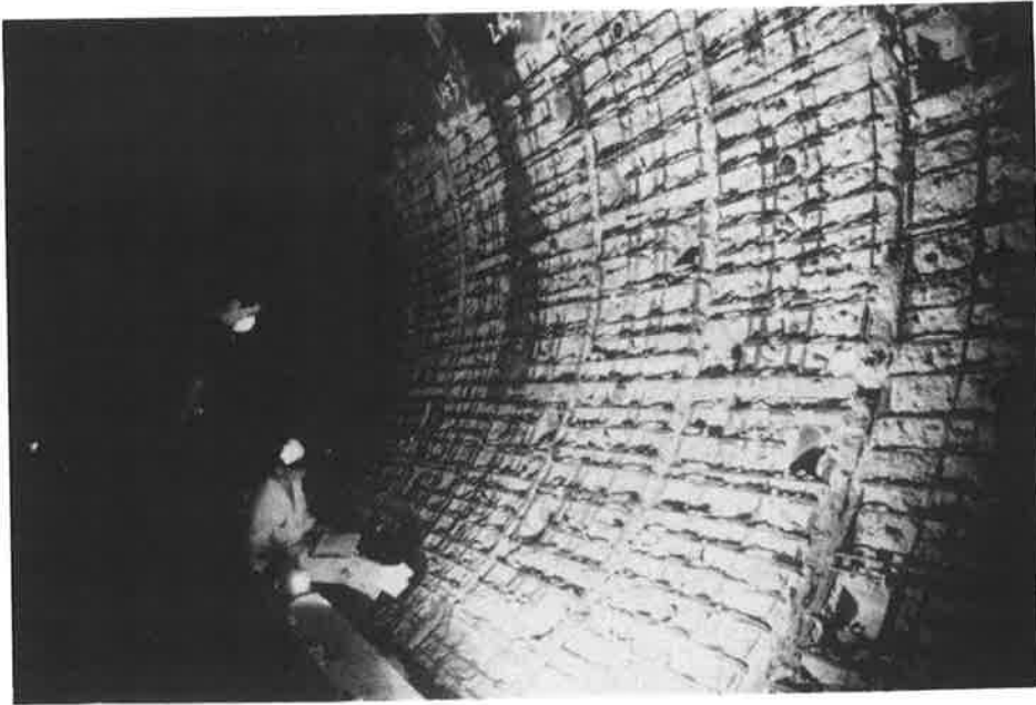
Fig. 7 Tunnel Lining after Hydrodemolition
