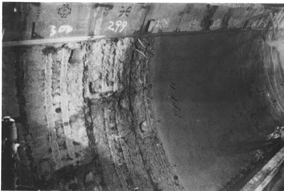
Fig. 9 Tunnel Lining after Shotcreting
