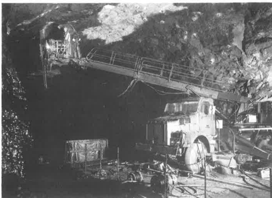
Figur 3 Endast en mindre del av taket hade ej varit i kontakt med oljan. A minor part of the roof had not been in contact with the oil.
