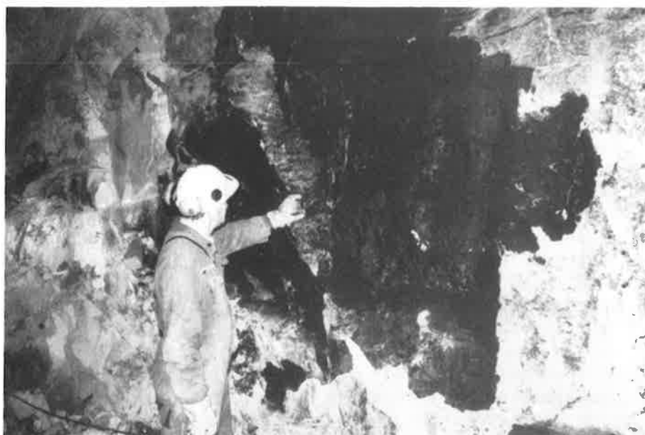
Figur 4 Brottytorna bakom block som lossnat var täckta med olja som trängt in i sprickor och reducerat sprickornas friktionsegenskaper. The rock surface behind loose rock were covered with oil which had filled open joints and reduced the friction.
