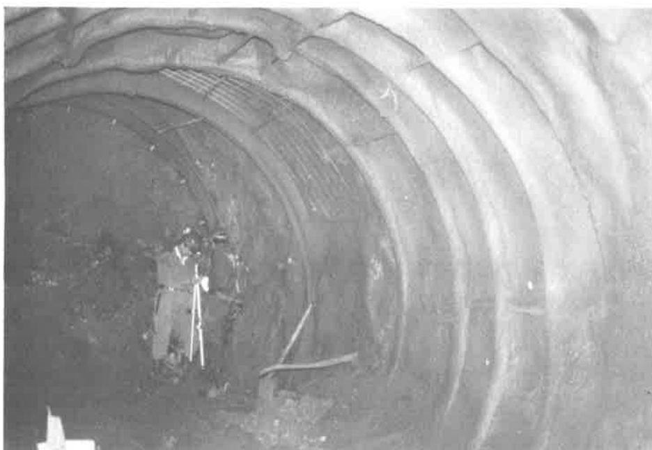
Figur 4 Avslutningsvis sprutades tunneln med ca 10 sprutbetong. Finally, a 10 cm thick lining was performed in shotcrete.
