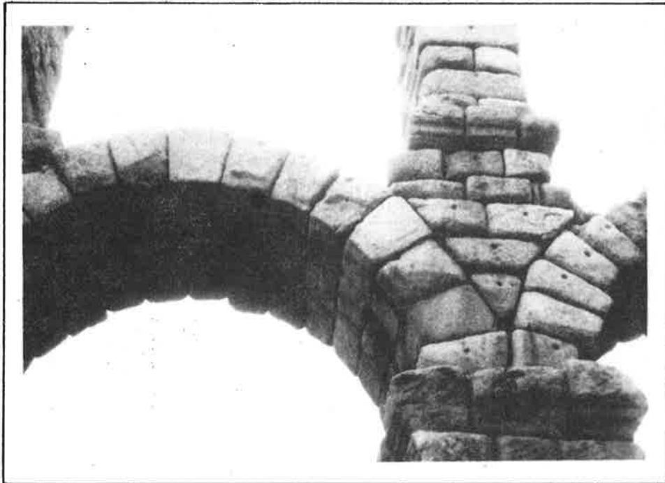
Figure 1. The importance of joint properties is illustrated by a classical Roman arch (Segovia, Spain).
