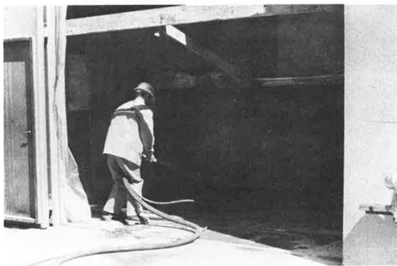
Operator in shotcreting position .
